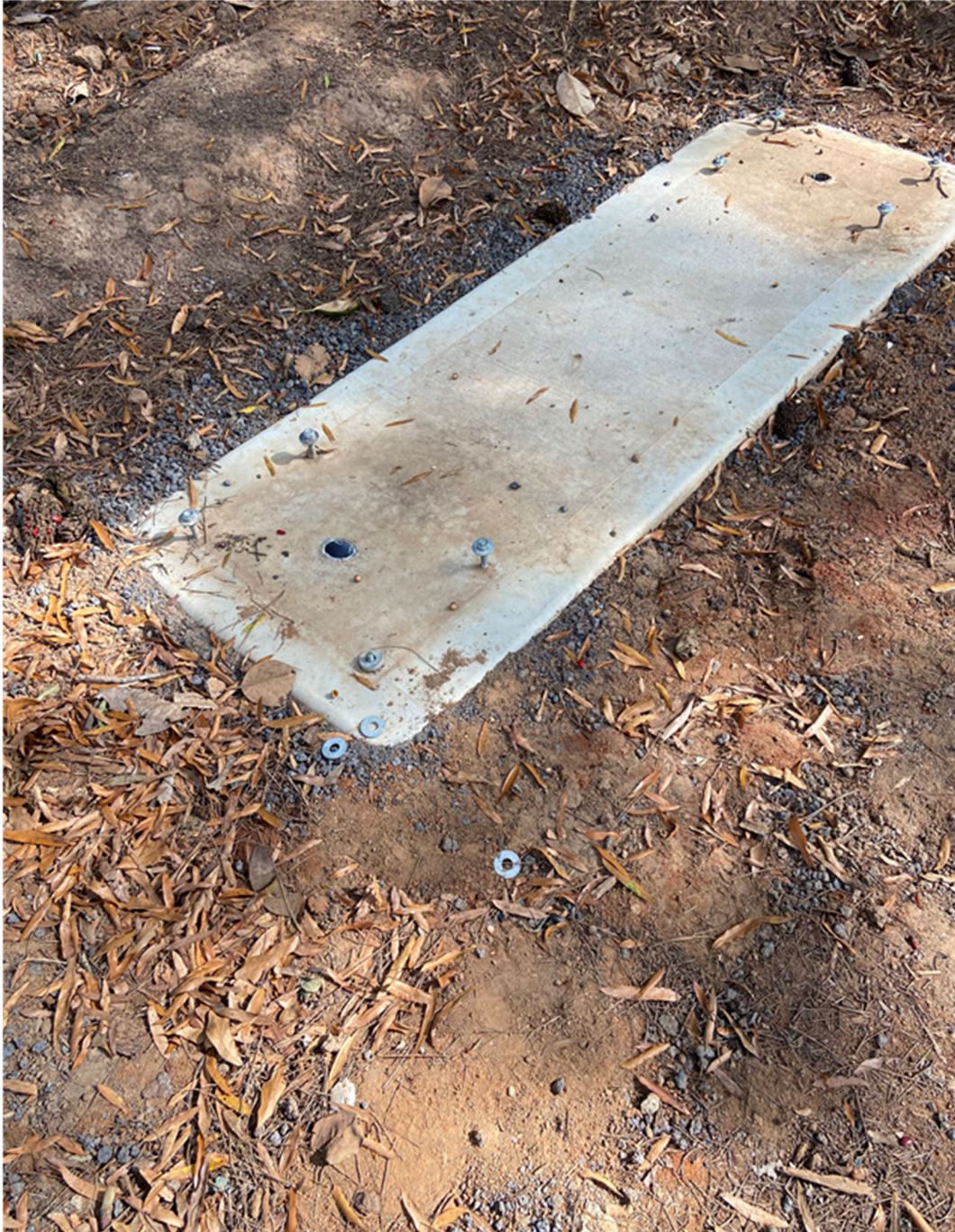
Photo of concrete slab - current
